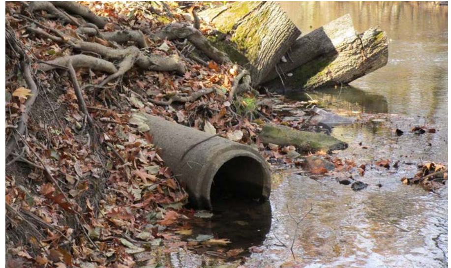
Stormwater discharge to the Pascack Brook in Hillsdale, NJ (Photo Credit: Rutgers Cooperative Extension)
