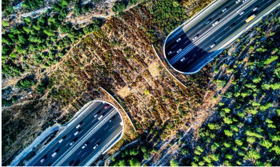
Wildlife crossings provide safe corridors for animals to cross human-created barriers, such as highways.
