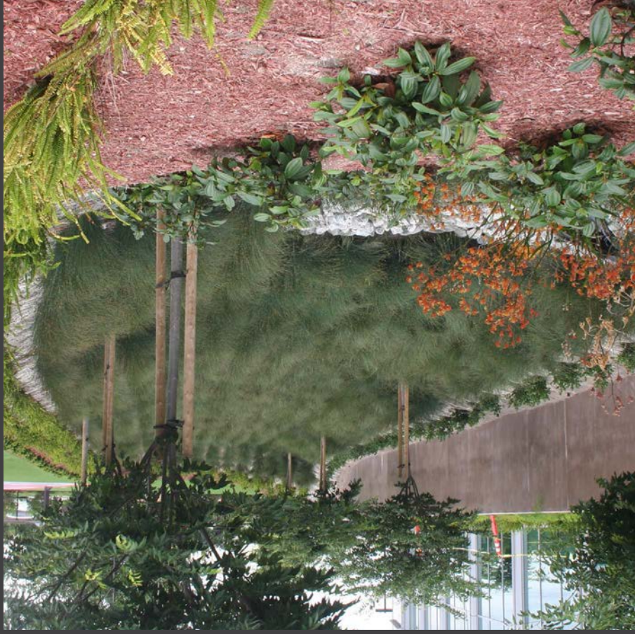
Bioswales allow water to move away from infrastructure or other sensitive areas, while also providing infiltration and pleasing aesthetics. (Photo Credit: Rutgers Cooperative Extension)
