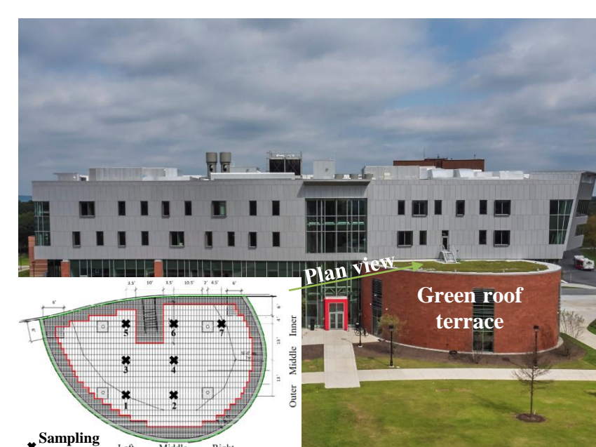
Figure 3. Green roof of the Richard Weeks Hall of Engineering at Rutgers
