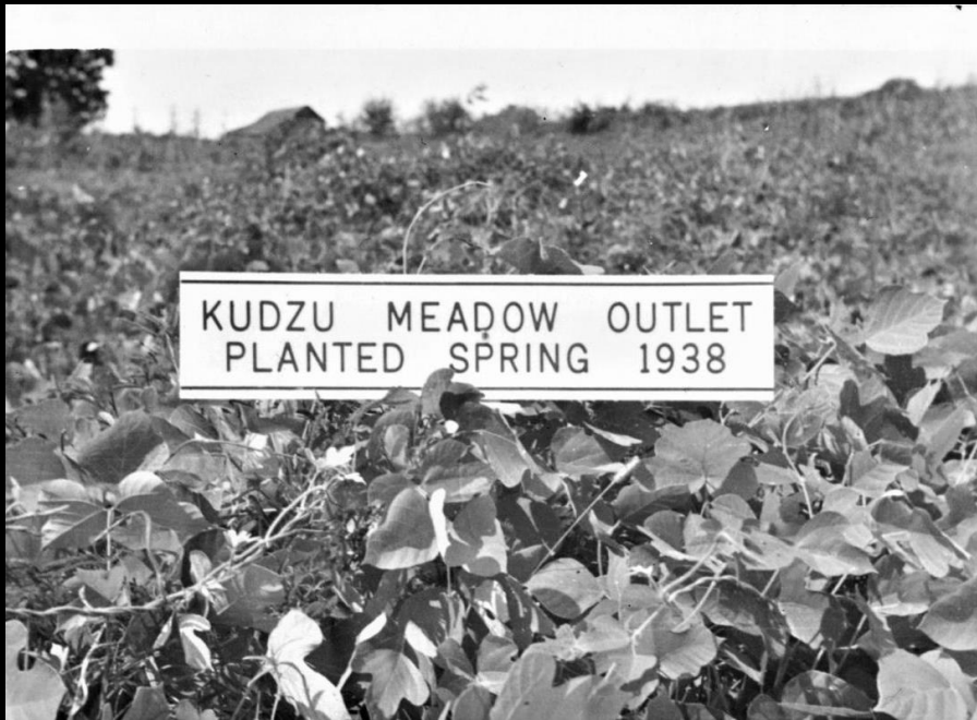
CCC Soil Erosion Project
