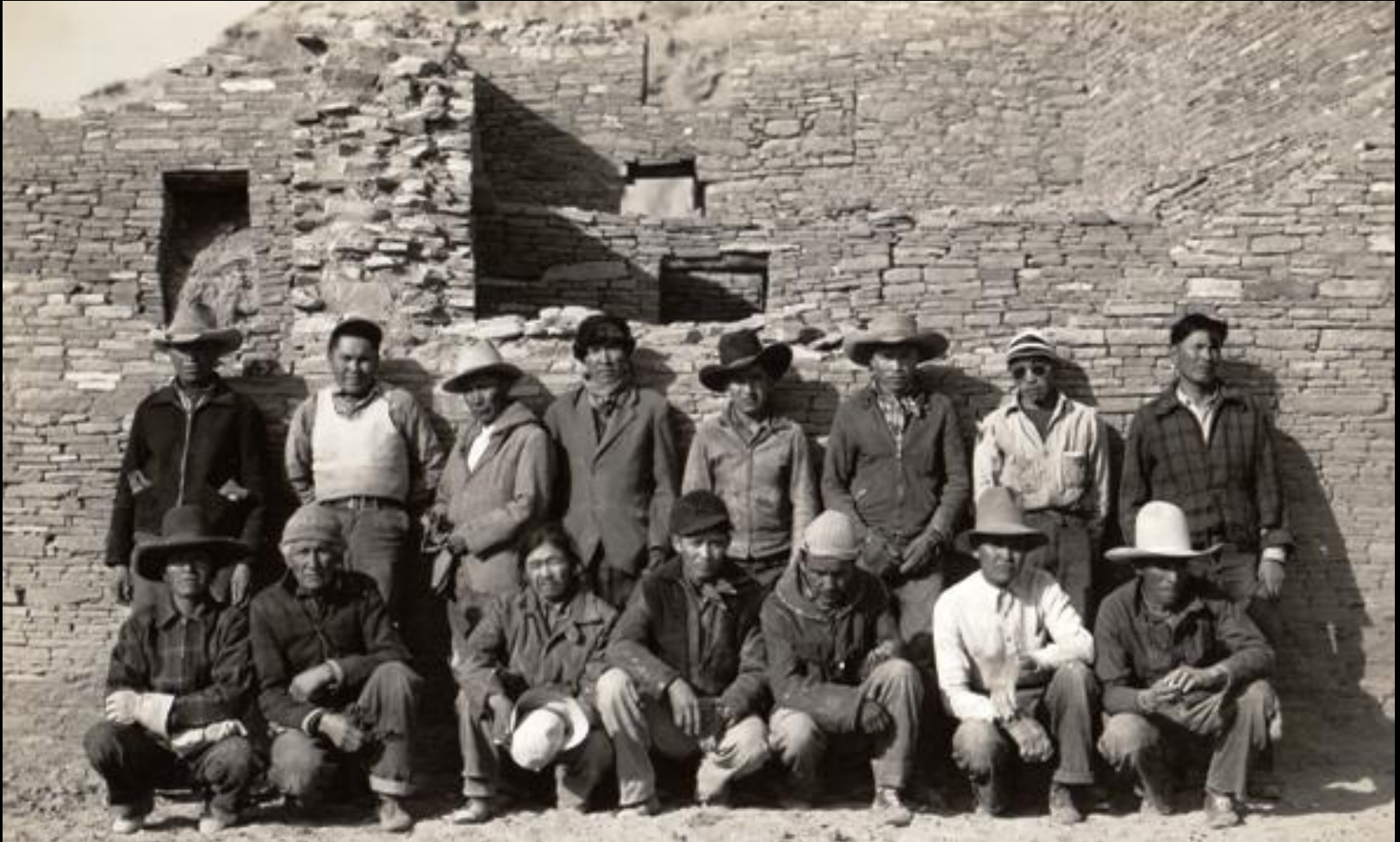
Navajo Enrollees Working in Chaco Canyon National Monument, 1938
