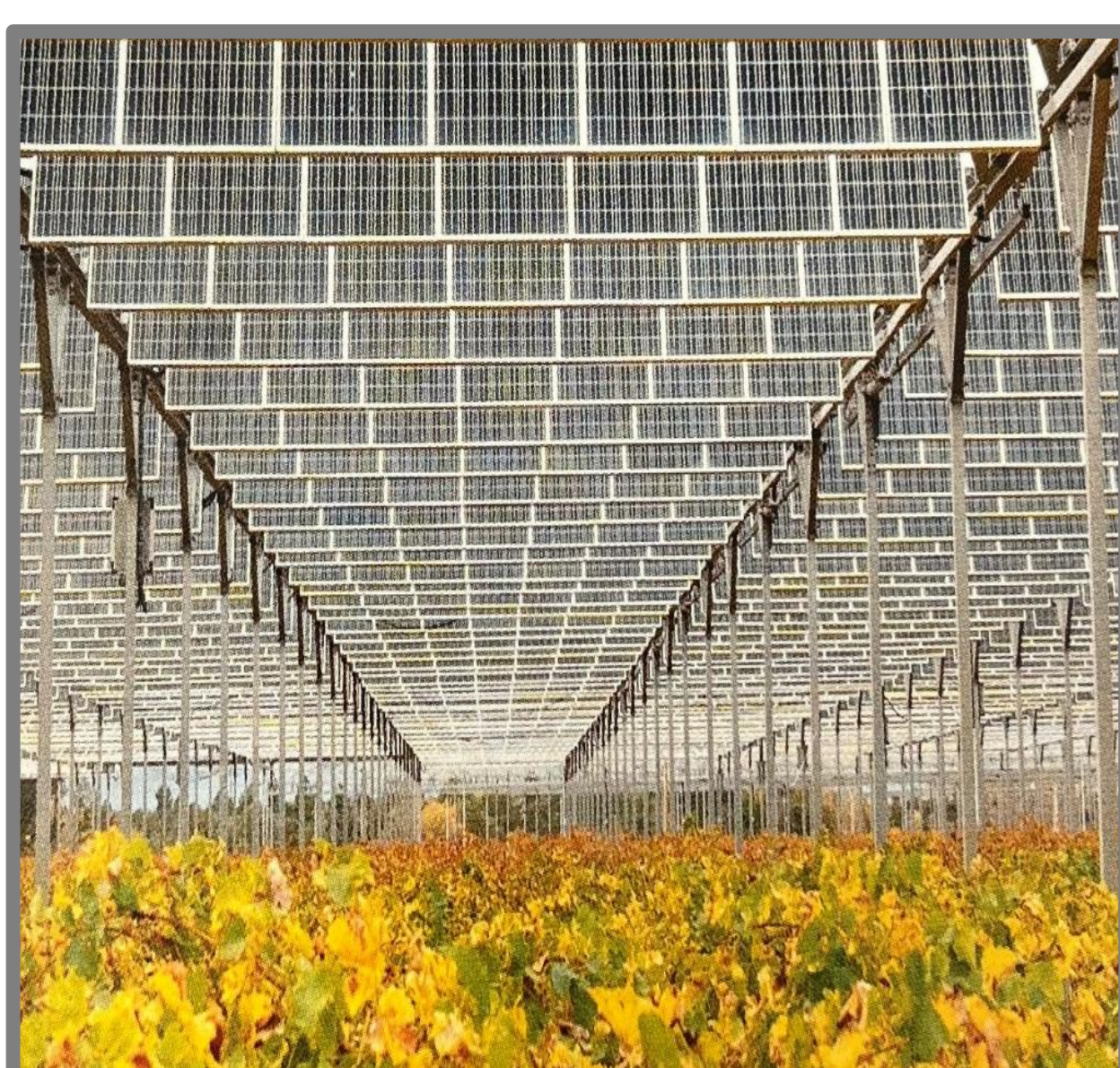
A single-axis tracking array raised above crops. Image from Optimum Tracker.
