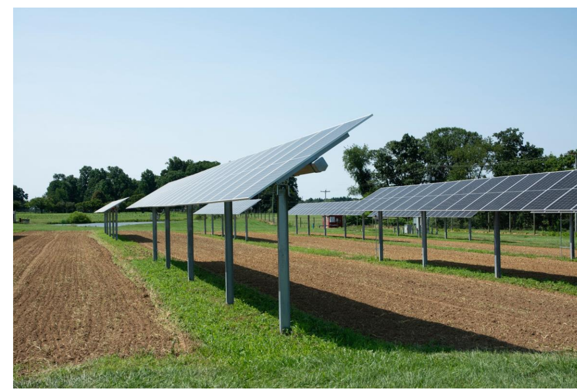
Site prepped for sowing grass
