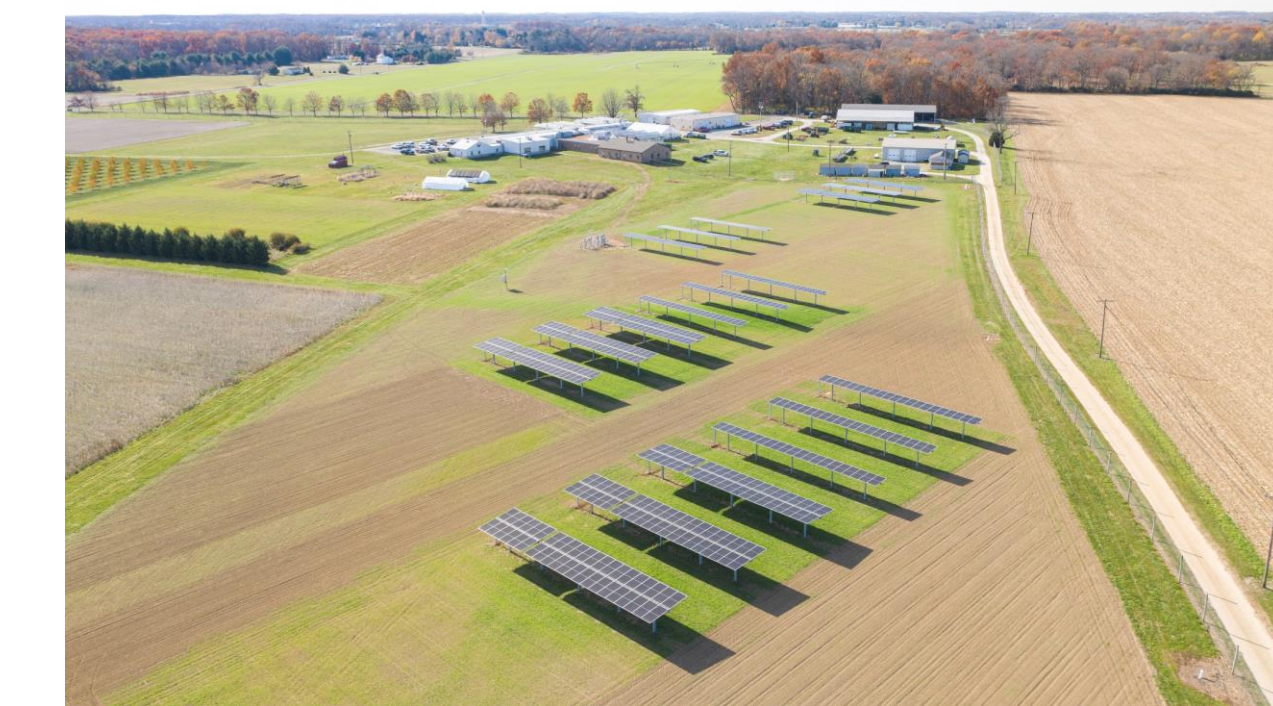
Site after installation of the solar panels
