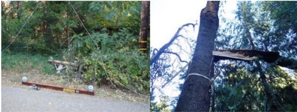
Figure 1. Foresthill, Placer County. Pole, cross-arm and conductor damaged by split tree.
